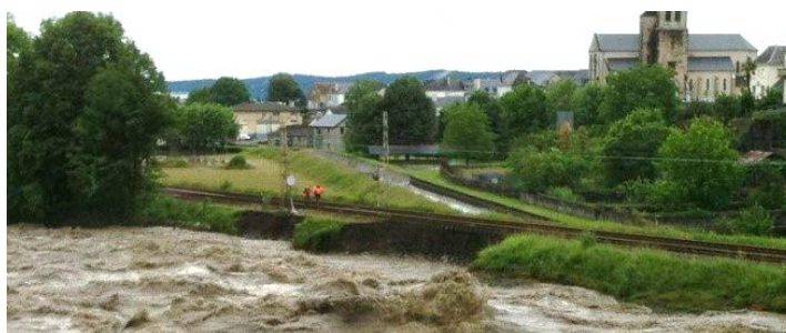
Figure 2. A picture of the railway line, on 18 th June 2013 (photo credit : SNCF)
